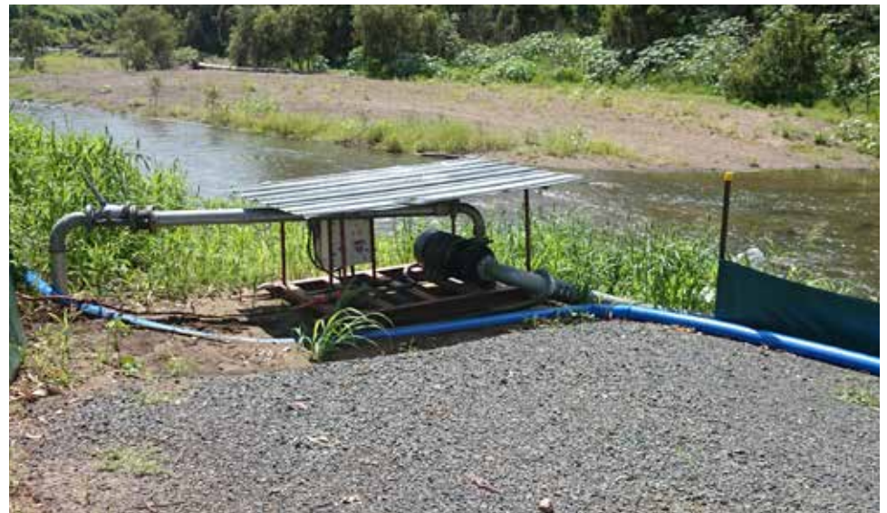
Ease of access to irrigation equipment in the event of river water rising can be considered as part of riparian works at each site
