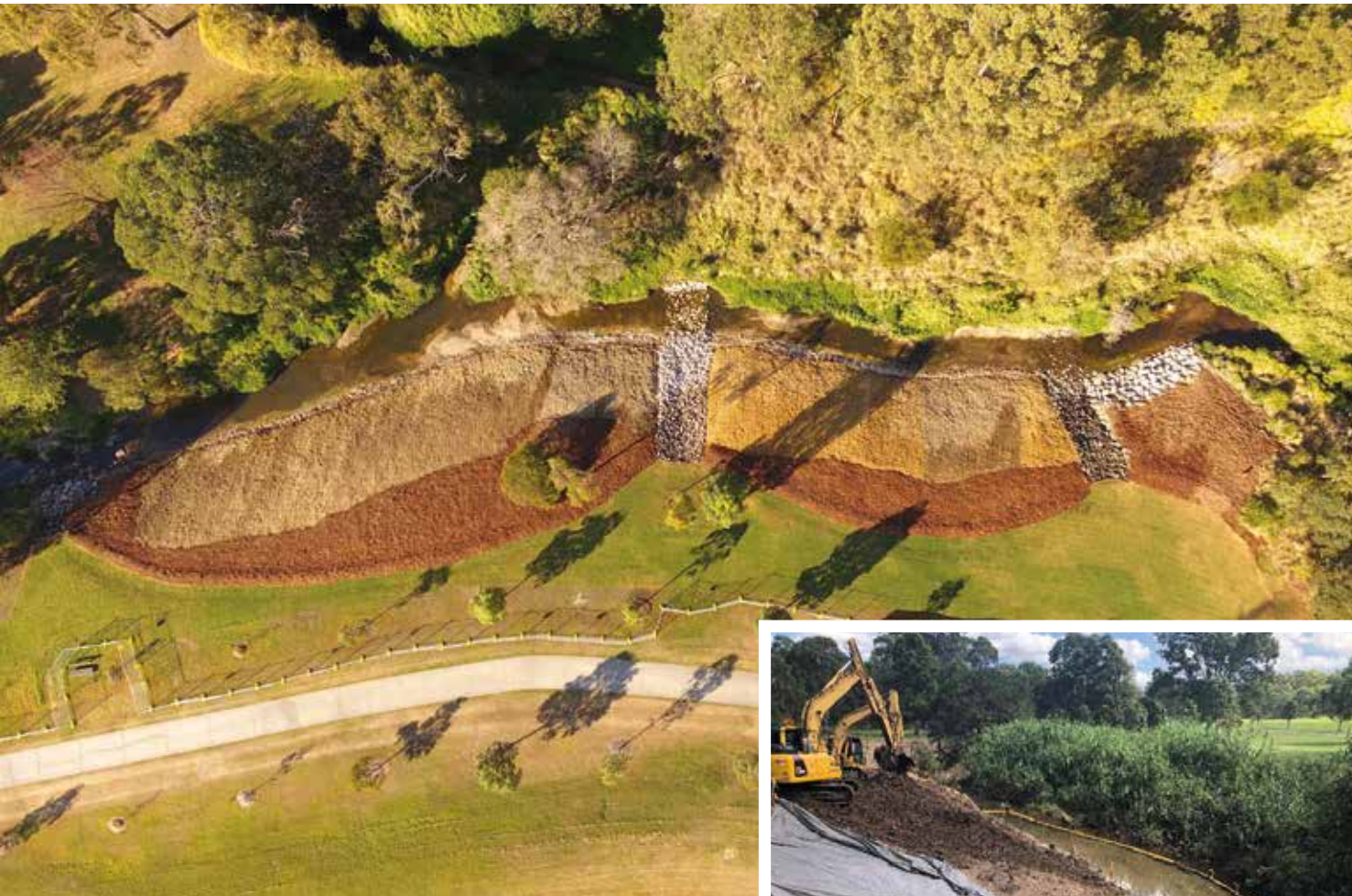
Downfall Creek Restoration Project – During construction and after
